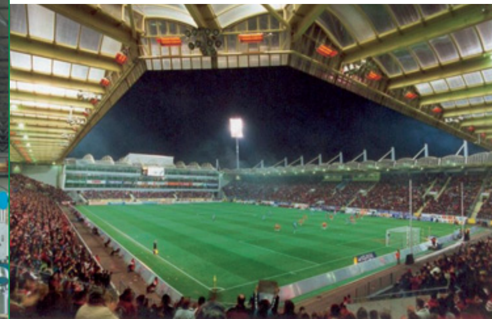
Heating of grandstands
