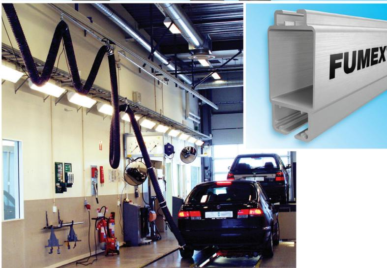
*The Fumex range also includes fans, accessories and control devices suitable for exhaust extractors*
